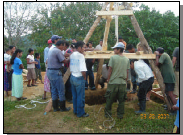
The well and caisson-lowering tripod is inspected
